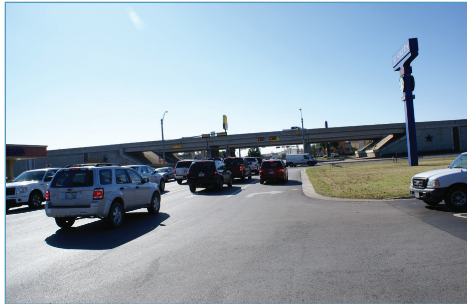
Hasler Boulevard traffic conditions at SH 71 on a weekday off-peak period
